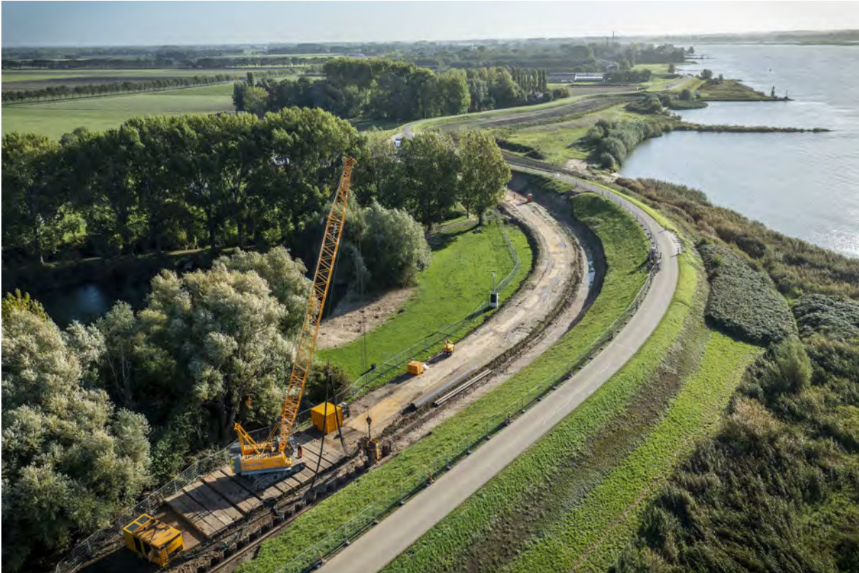
On our Gorinchem-Waardenburg (GoWa) dyke reinforcement project, we are using an electric wire crane. This 80-tonne crawler crane has a 37-metre boom (max. 58m) and operates completely emissions free
