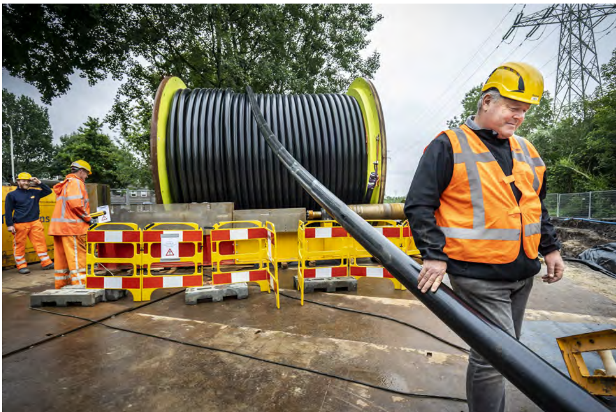
Maintenance of energy networks by Heijmans Cables and Pipelines
