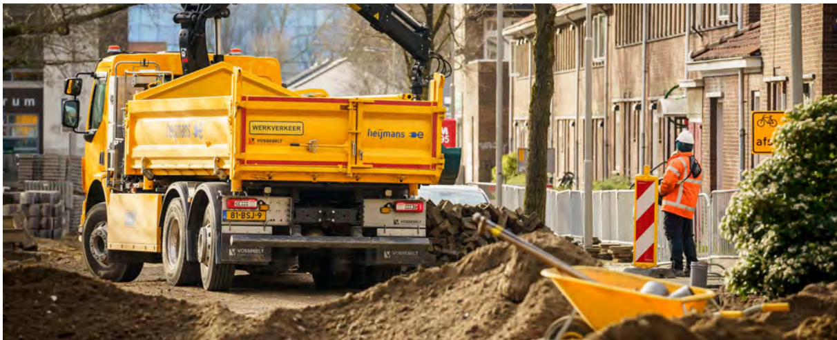
Electric truck at a project in Amsterdam
